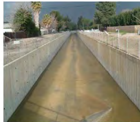
Looking northeast down the Arroyo Calabasas at parcel E
